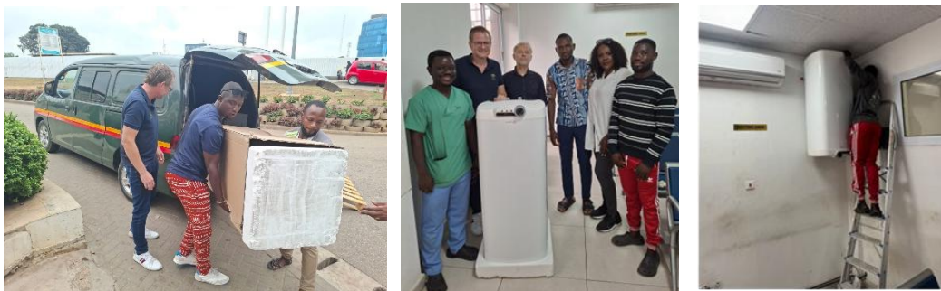
(Test-Installation at Ridge Hospital, Accra)
